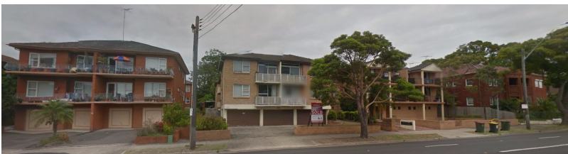
Figure 8 - Opposite site along Harrow Road
