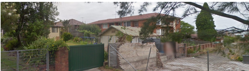
Figure 15 - View of rear of Frederick Street properties
